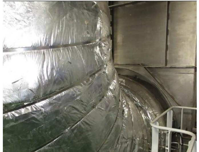
Scrubber installation-exhaust connection
